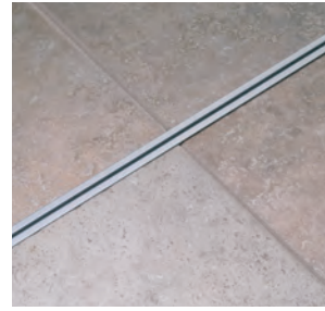
↑ Single rebated track set directly into tiling.
