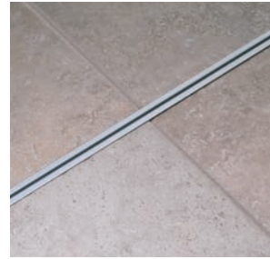
↑ Single rebated track set directly into tiling.
